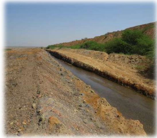
Catch drain around the external Dumps
