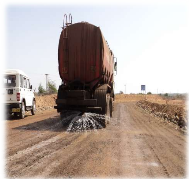
Water sprinkling system provided to check dust emissions at haul road.
