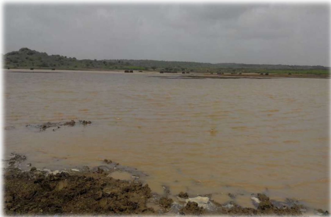
Dam preparation at Mata-No-Madh village
