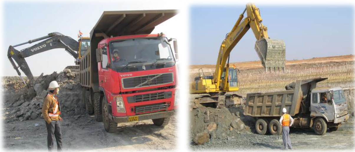
Workers using PPE's
