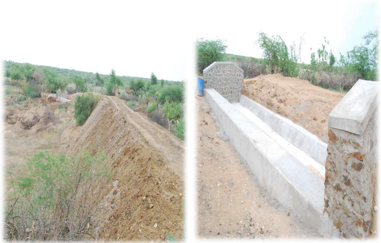
Dam preparation at Lifri village
