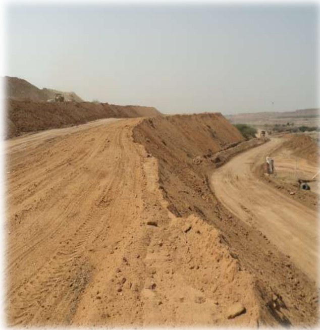
In pit backfilled area and Plantation/reclamation work going on
