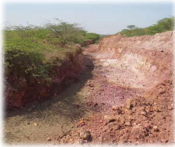
Catch drain around the external Dumps
