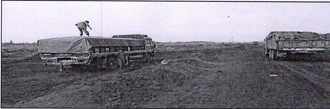
Photograph of truck covered with tarpaulin is shown below.
