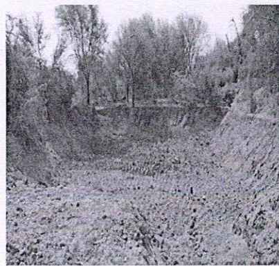
Silting pond preparation
